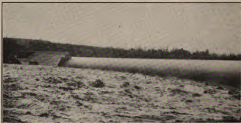
Fig. 14.—The flood passing the Scioto river storage dam, afternoon of March 25, 1913.
